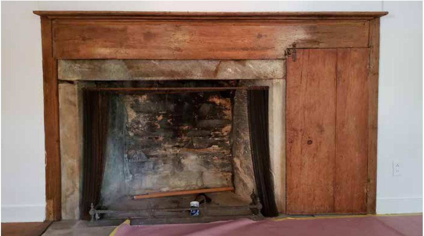
Original fireplace in the MHS Rocking Stone cottage
